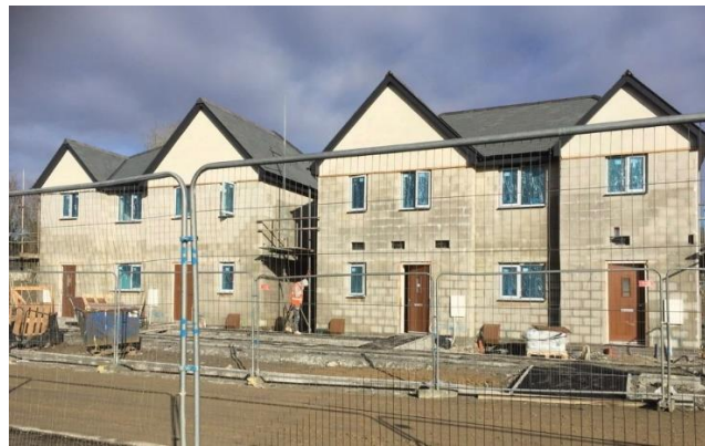
Fig. 1 Crapstone, Devon. Under construction.
