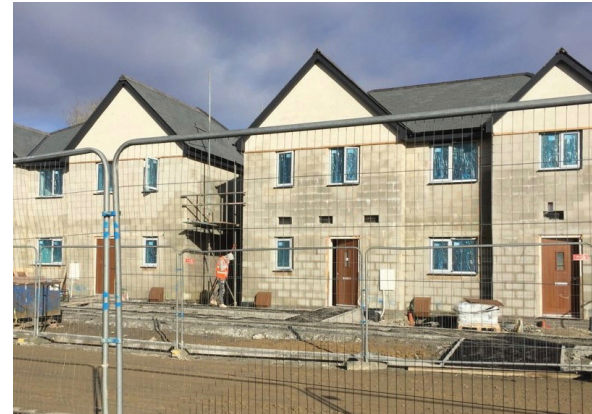
Construction at Crapstone
