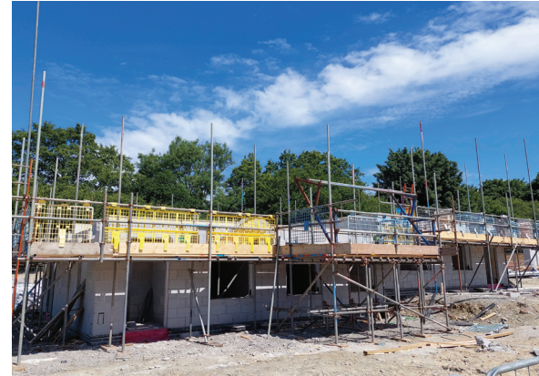
Construction at Crapstone
